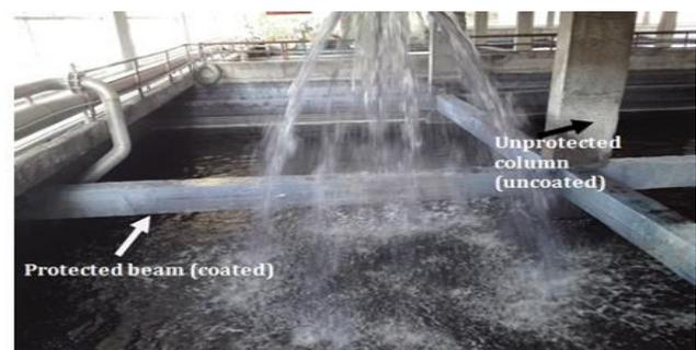
**Fig. 3:** Protected beam unprotected column.
